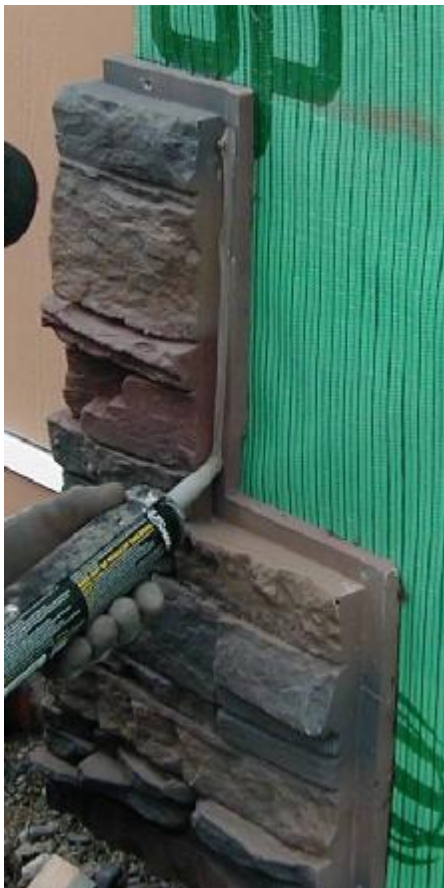
Apply caulk to all positive lips and screw holes.
