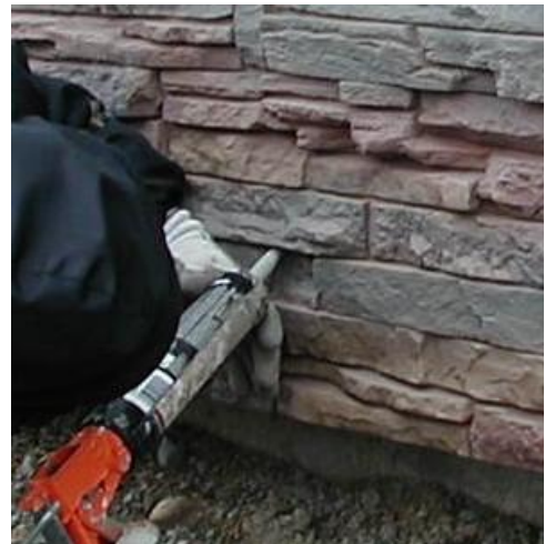
Apply caulk to all positive lips and screw holes.
